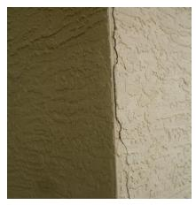
• Repair: Stucco cracks in various places should be sealed. This signifies that the home has experienced typical settling.
