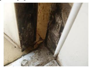
• **Repair:** The hole at the back porch wall needs sealing.
