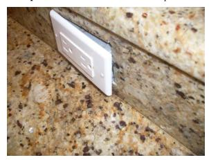
**Repair:** A broken outlet cover was found in the office.
