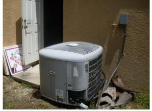
• **Repair:** The AC drain should be extended away from the foundation.
