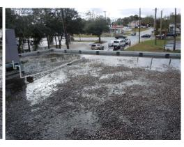
• Repair: The tar has dried and cracked and has allowed many leaks with water damage to the roof over the drive thru.
